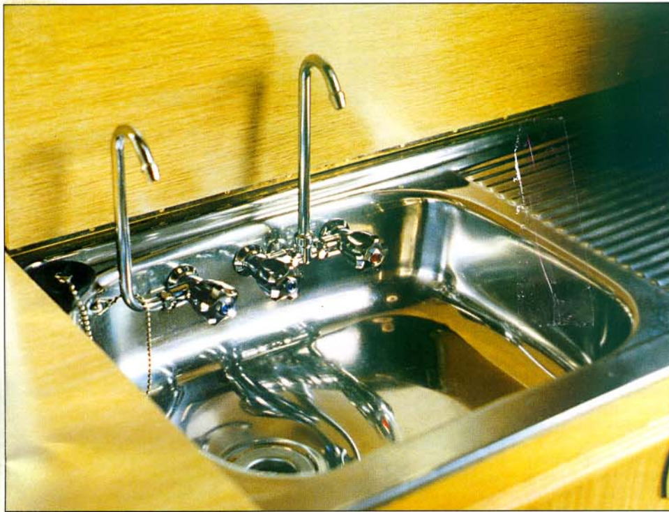
The completed job. If you look very closely, the blanking plug can be seen behind the mixer faucet.
